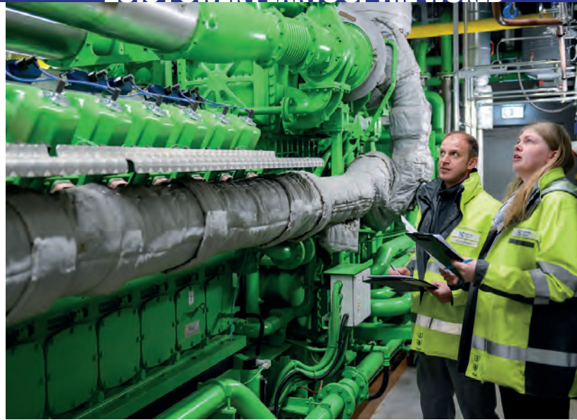
Jenbacher Type 6 gas engines from INNIO are used at HanseWerk Natur's CHP plant.
